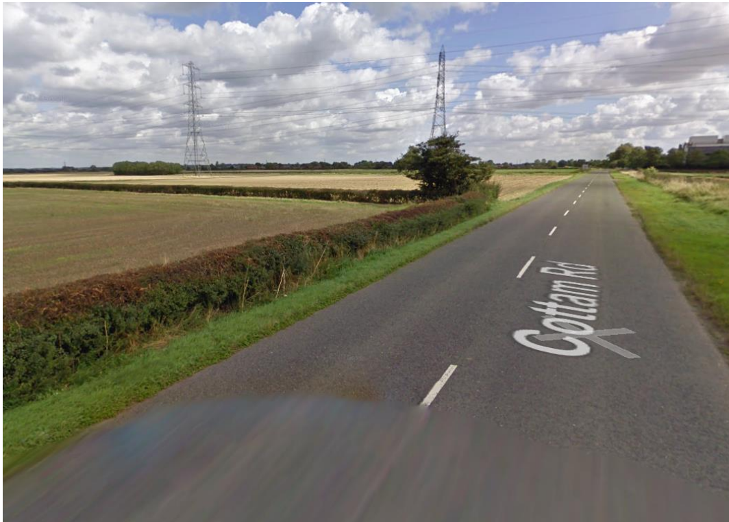
Figure 37: Cottam Road North Access Existing Layout Street View
